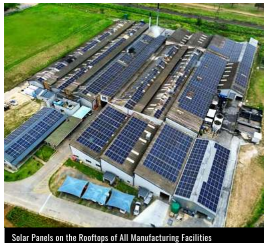
Solar Panels on the Rooftops of All Manufacturing Facilities
