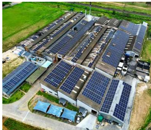
Solar Panels on the Rooftops of All Manufacturing Facilities
